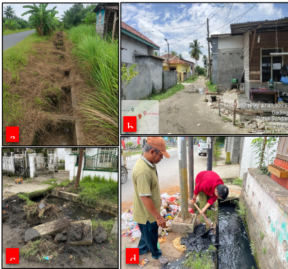
Figure 1. a) The existing condition of the Tanjungbalai City Drainage is covered with sediment and wild plants; b) drainage in the residential environment of one of the sub-districts in Tanjungbalai City where several channels have not been connected and the environment is often flooded; c) condition of damaged stone pairing channels; d) Drainage conditions with water runoff mixed with domestic waste increase the potential for groundwater pollution and surrounding water bodies (Source: Tanjungbalai City PUTR Office Documentation, 2024-2025)
